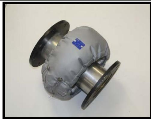
Step 6 – Flange blanket shaped. Remove spare wire. Fasten blanket by wrapping draw cord wire around rivets.
